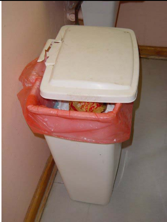
Broken pedal bin for HCRW in sluice room
